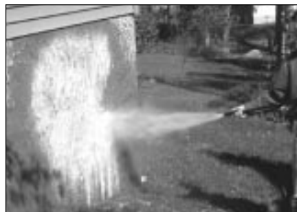
Figure 6 - Detergent application
